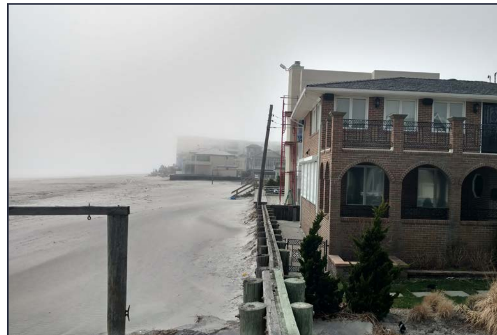
Beachfront Construction, Longport
