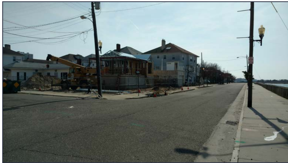
Ongoing Recovery Construction, Ventnor City
