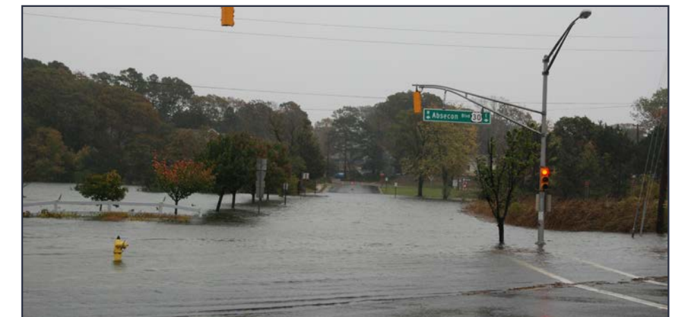
White Horse Pike flooded Photo Credit: Atlantic County
