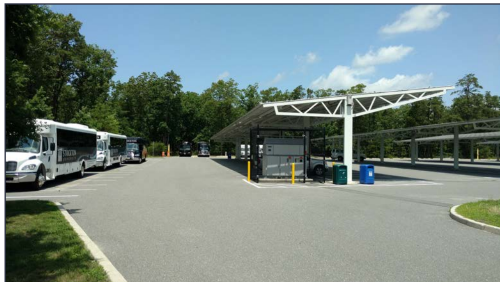
Solar Canopy seen at Stockton University in Galloway Township
