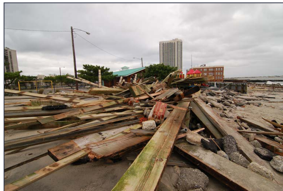
County Damage from Superstorm Sandy Photo Credit: Atlantic County
