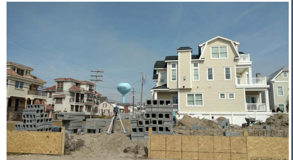
New Home Site, Longport
