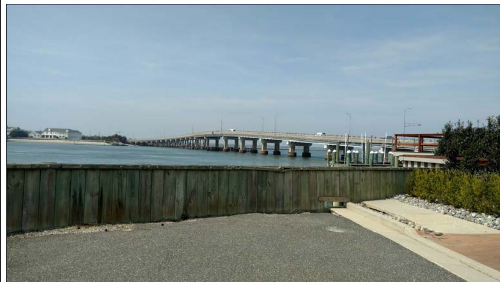
JFK Memorial Bridge, Longport
